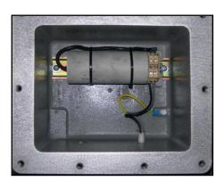
Fig. 1.3 View of capacitor fitted in dedicated box (single phase voltage)
